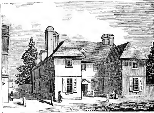
THE OLD SLATE-ROOF HOUSE.
